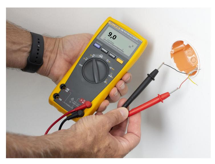
A cavity wall box with Ø 68 mm and 60 mm (diagonal) device screw spacing is ideal for wall reader flush mounting. A mounting depth of 35 mm is sufficient.
