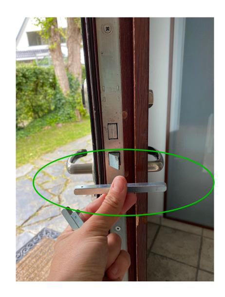
XLOCK TIP: This is a very important step! As thie square shaft is the part that connects the front and back panel. Check page 23 for more detailed pictures of the installed square shaft.
