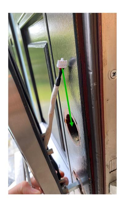
! The cable needs to get through this hole in the mortize lock to connect with the back panel!
