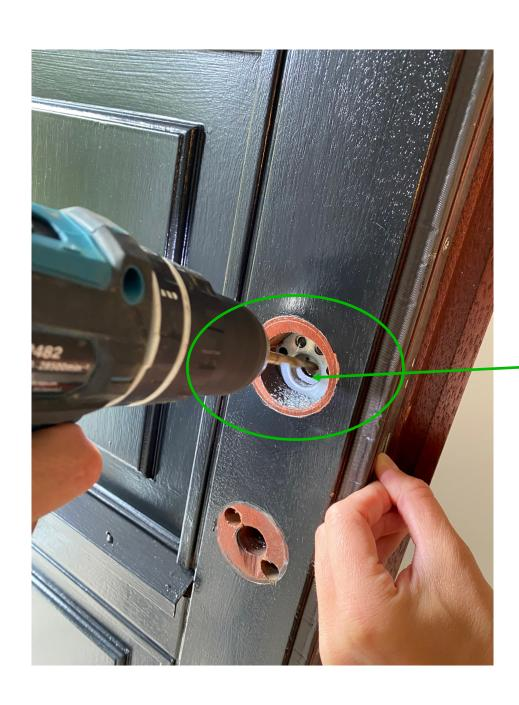
In some cases you might need to drill a bigger hole in the mortize lock to fit the cable through.
