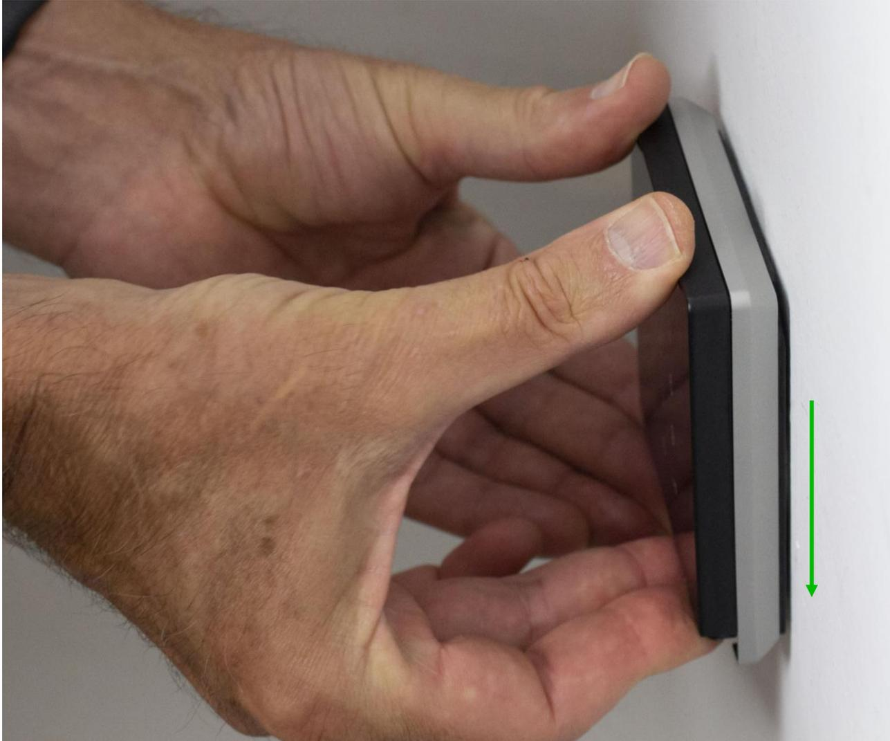
Push the wall reader from top to bottom until it clicks into place on the flush-mounted mounting frame. Then press the locking bar until it clicks into place - CLICK.
