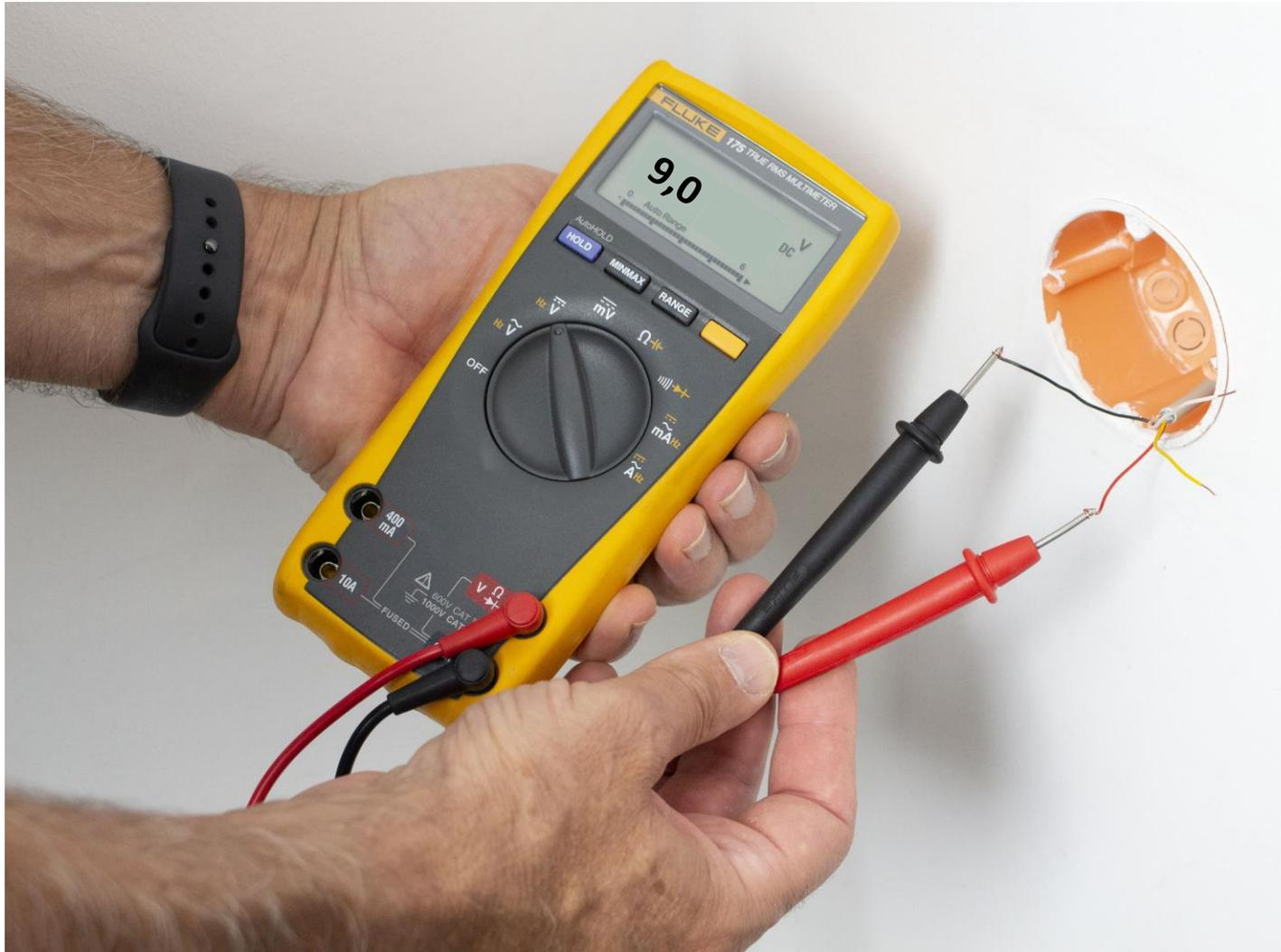
A cavity wall box with  $\varnothing$  68 mm and 60 mm (diagonal) device screw spacing is ideal for wall reader flush mounting. A mounting depth of 35 mm is sufficient.
